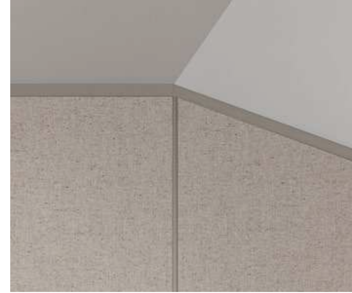
Detail of shaped panel for sloped ceiling
